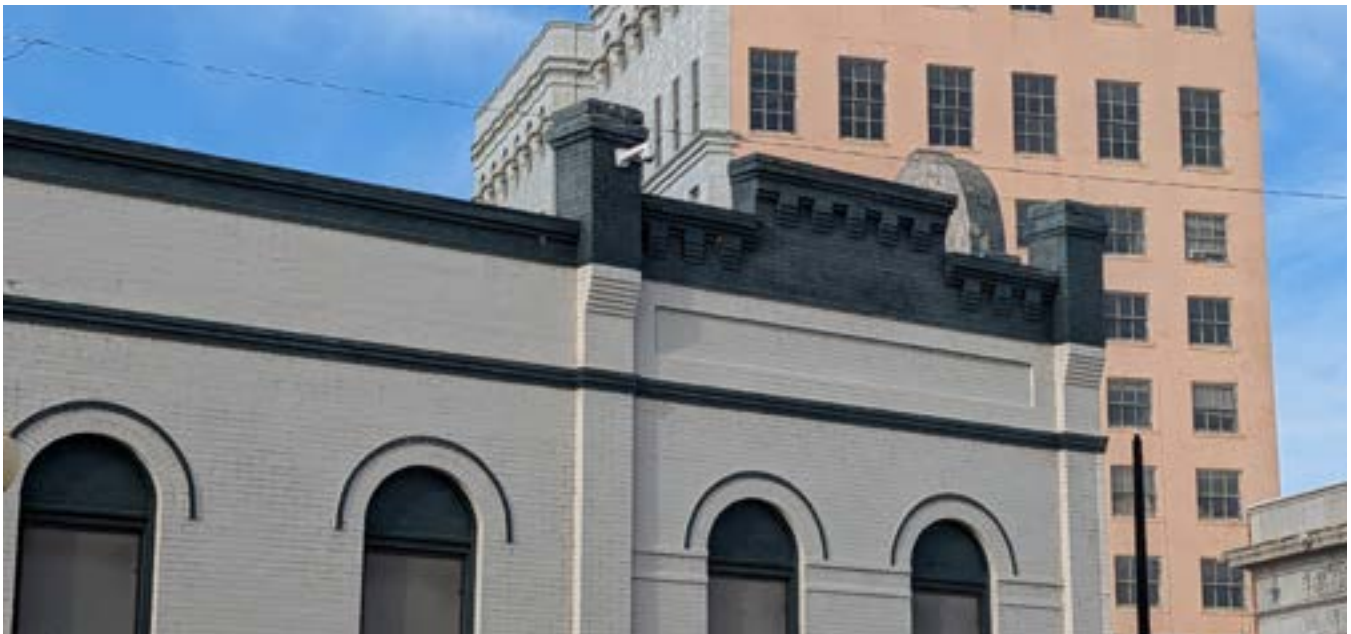
Figure 3.11. The installation of equipment and hardware to a building can negatively impact its profile and appearance. The security camera mounted to the parapet on this Patton Street building is barely visible from the right-of-way.
