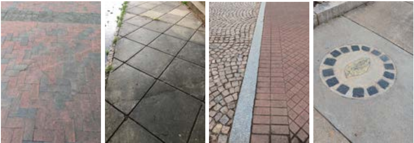
Figure 4.11. Some historic sidewalk materials and patterns found in the ARO include brick laid in a common bond pattern or a herringbone pattern, concrete scored in a diamond pattern. Tobacco leaves can also be found in OWE sidewalks.
