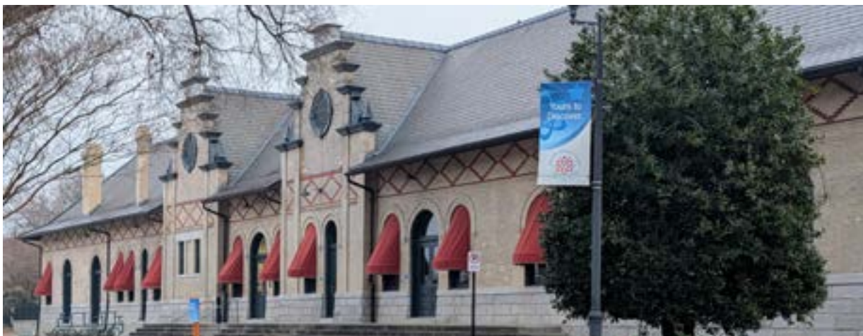
Figure 2.16. Awnings typically adorn commercial buildings, such as the row of canvas awnings in the upper left; the sign awning in the upper right; and the canvas awnings in the lower left. However, both metal and fabric awnings were applied to houses.
