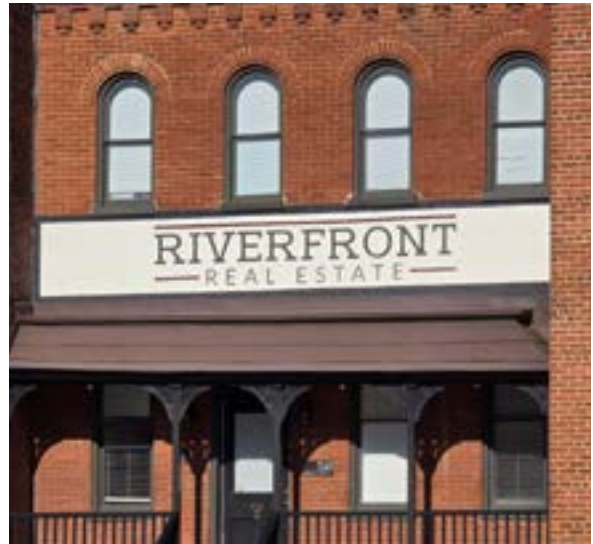
Figure 5.4. The colors of this painted Riverfront Real Estate sign complement the building materials and the colors of the building's trim.
