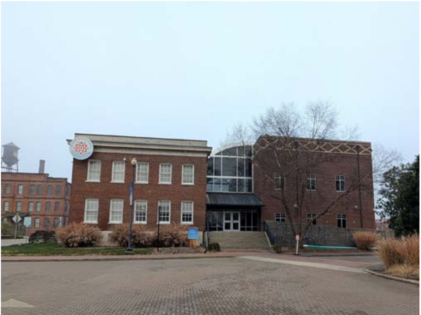
Figure 4.3. The Danville Science Center comprises two distinct structures: a modern addition on the right that mirrors the original building's setback and masonry (on the left), linked by a contemporary glass corridor to bridge the two styles.
