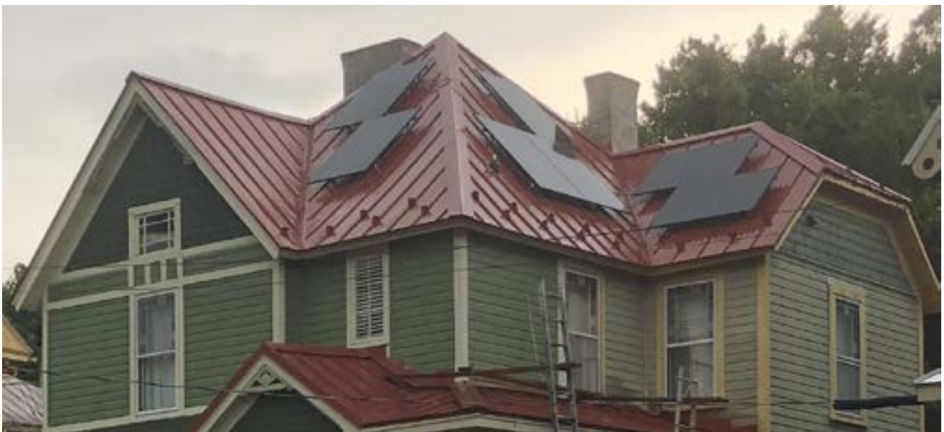
Figure 2.24. These solar panels have been placed on the front elevation of the house, are highly visible from the public right-of-way, do not match the color of the roof and thereby do not blend in with their background, and are not screened from view. This placement and treatment is highly discouraged.
