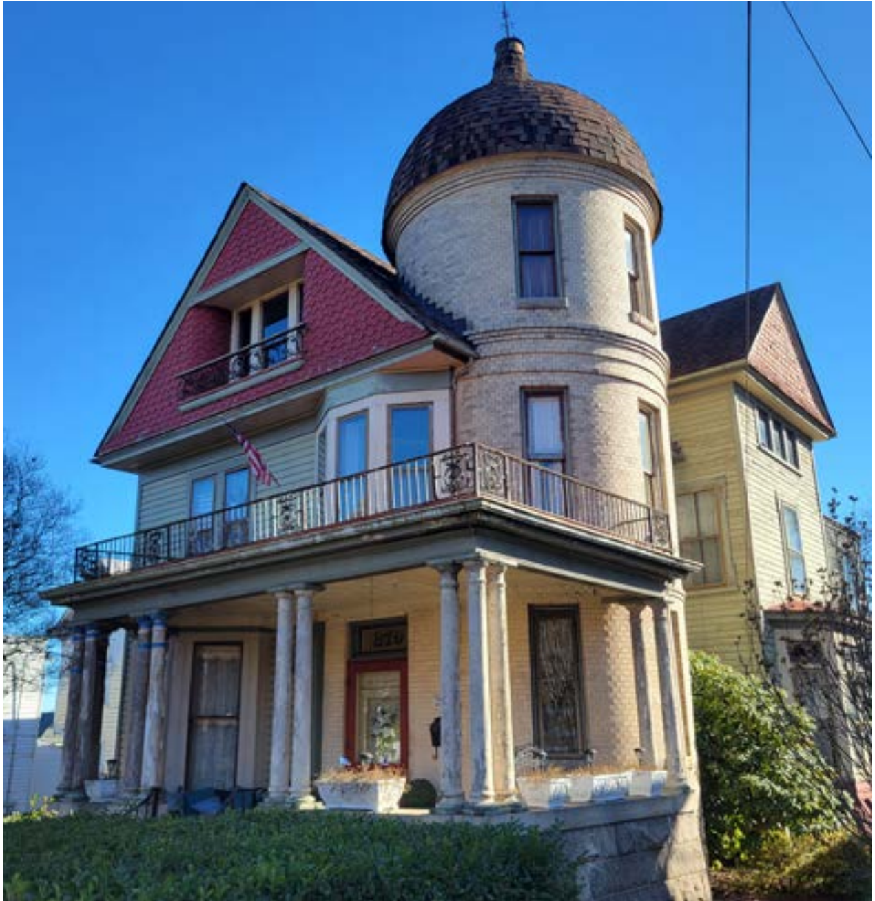
Figure 2.17. The R.B. Graham House, located at 879 Green Street, features double hung windows, bay windows at the front and side façades, and a stained glass window on the conical tower.
