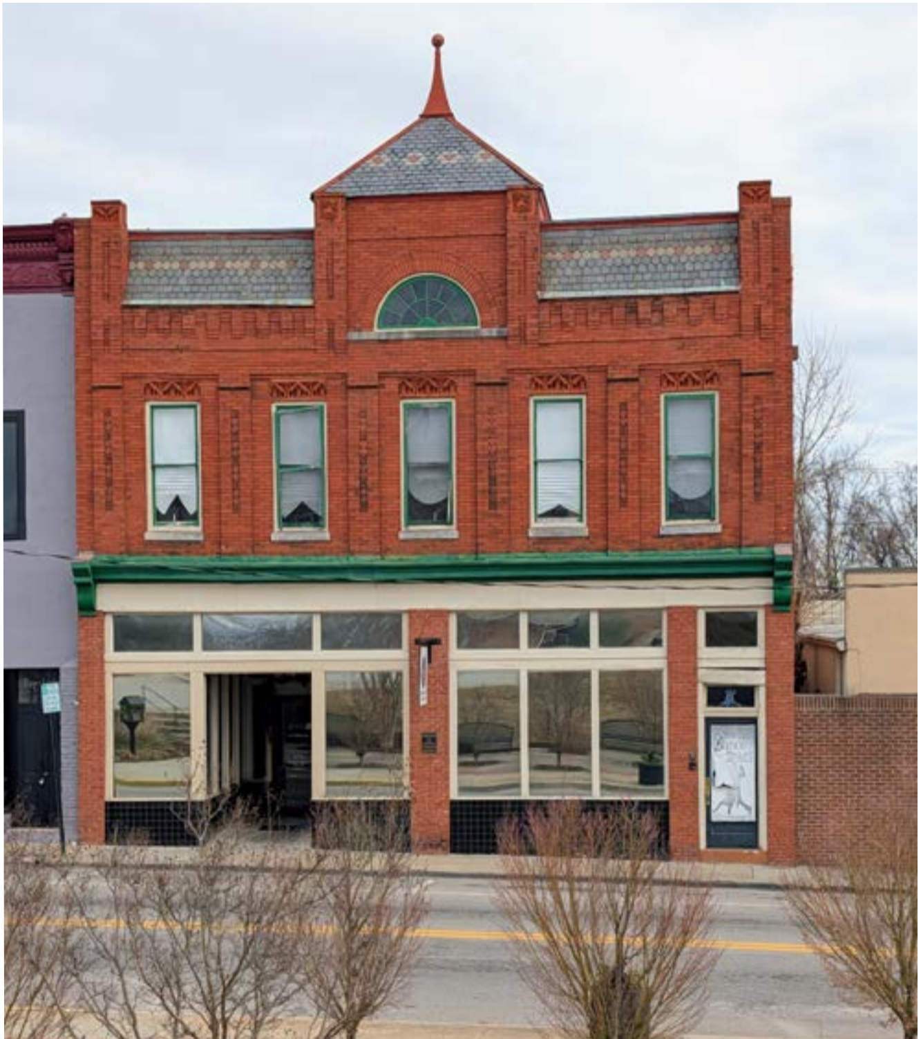
Figure 2.12. This classic commercial storefront system in the NMBD includes a base clad in ceramic tiles, large plate-glass and transom windows in a wood framing system, a recessed entry, and a decorative cornice.
