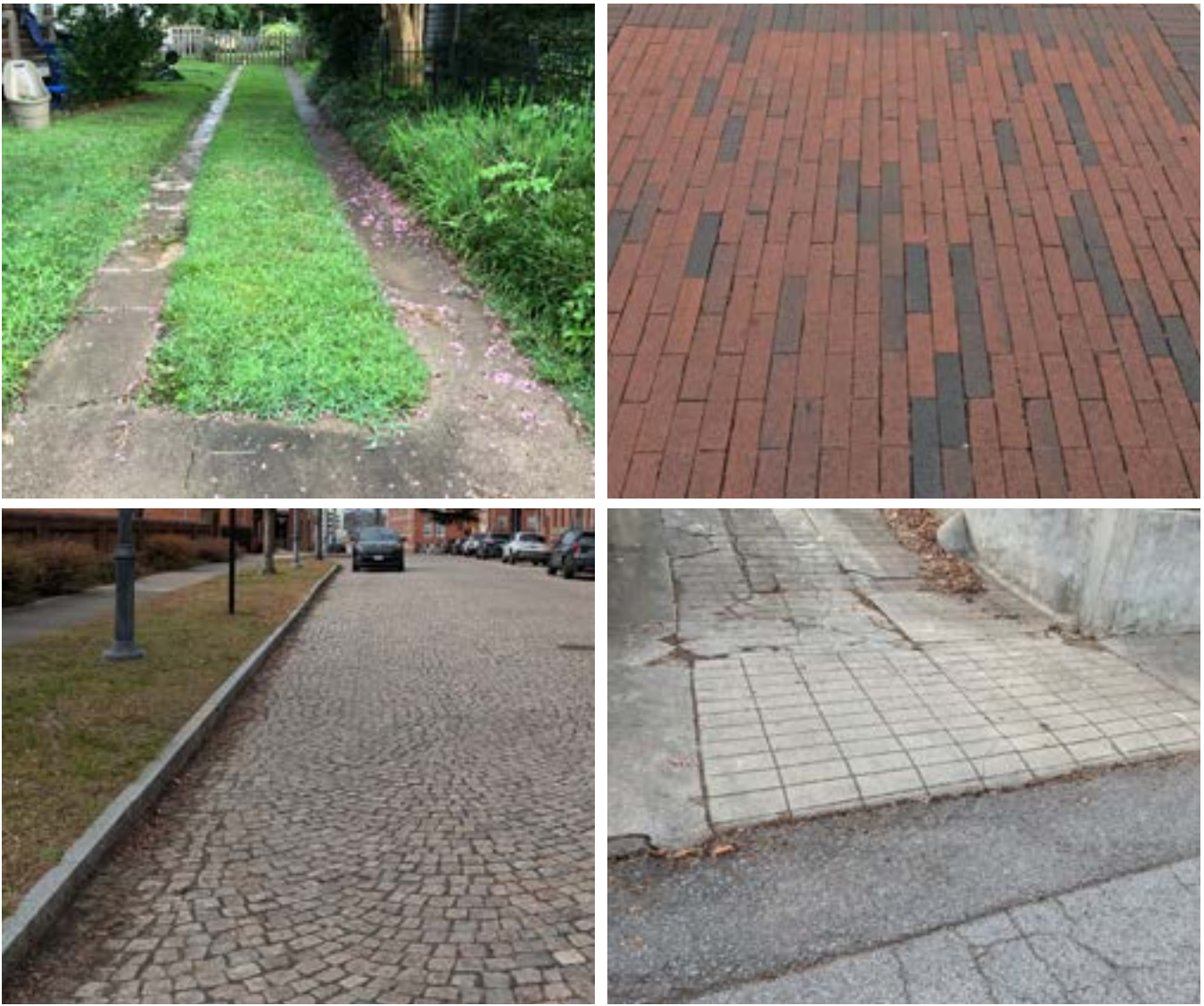
Figure 4.5. Historic driveways, driveway aprons, and curb materials should be preserved in place, repaired, or replaced in-kind.
