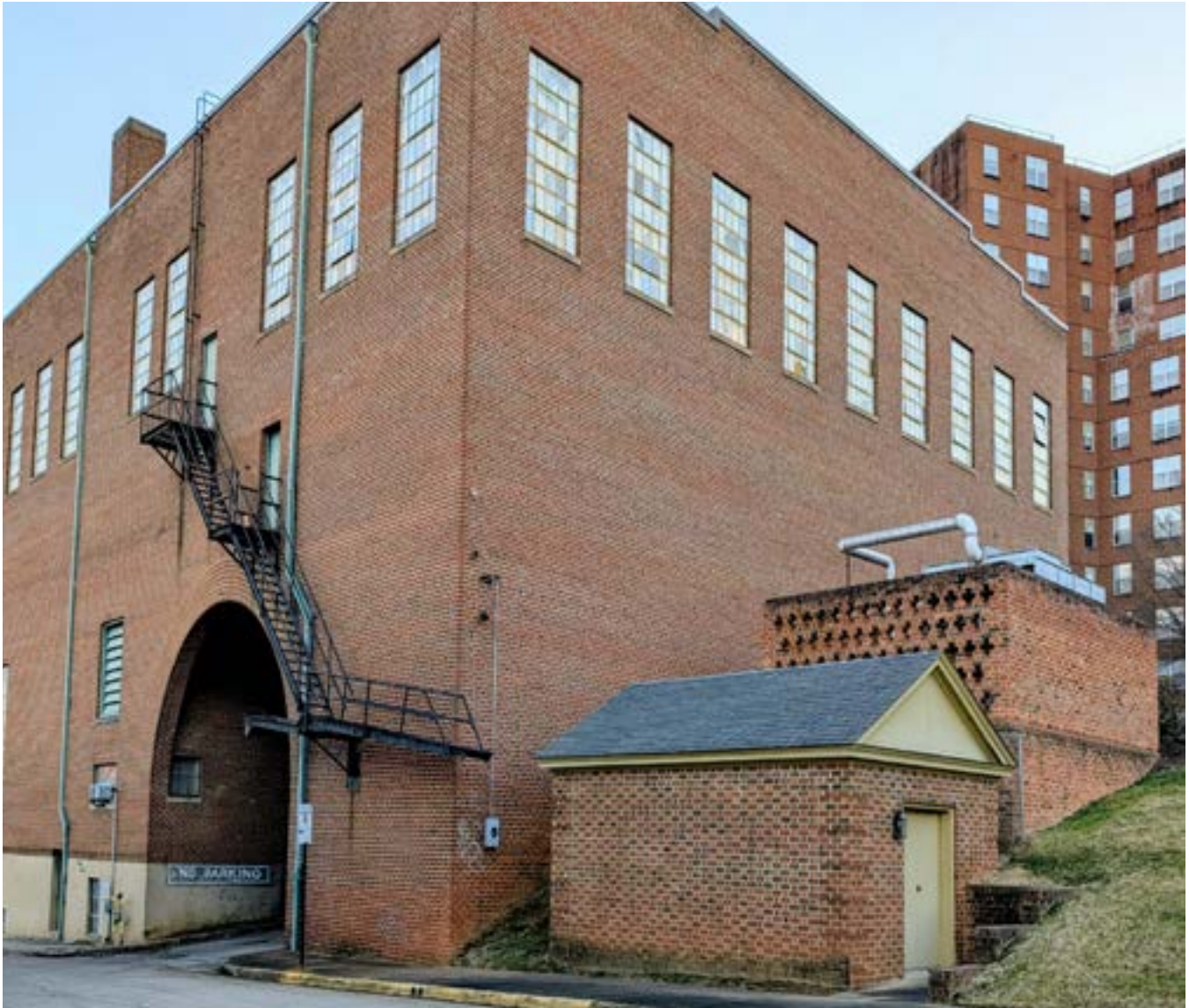
Figure 2.22. This Spring Street example serves as a model for screening utilitarian equipment by utilizing high-quality materials that complement the primary architecture.
