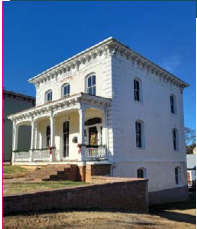
Figure 2.13. The home at 864 Pine Street boasts a decorative Italiante porch and low-slope roof adorned with intricate cornices.
