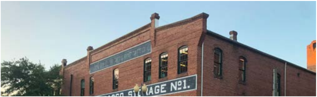
Figure 2.8. Late 19 th and early 20 th -century vernacular commercial buildings typically have flat roofs hidden behind parapets, which are vertical extensions of the façade. This building features a stepped parapet.
