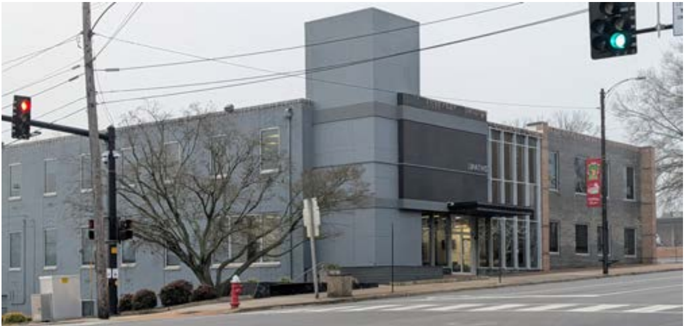
Figure 3.12. Located near the southern edge of the River District, Paths utilizes traditional masonry to harmonize with the historic architecture of Main Street.
