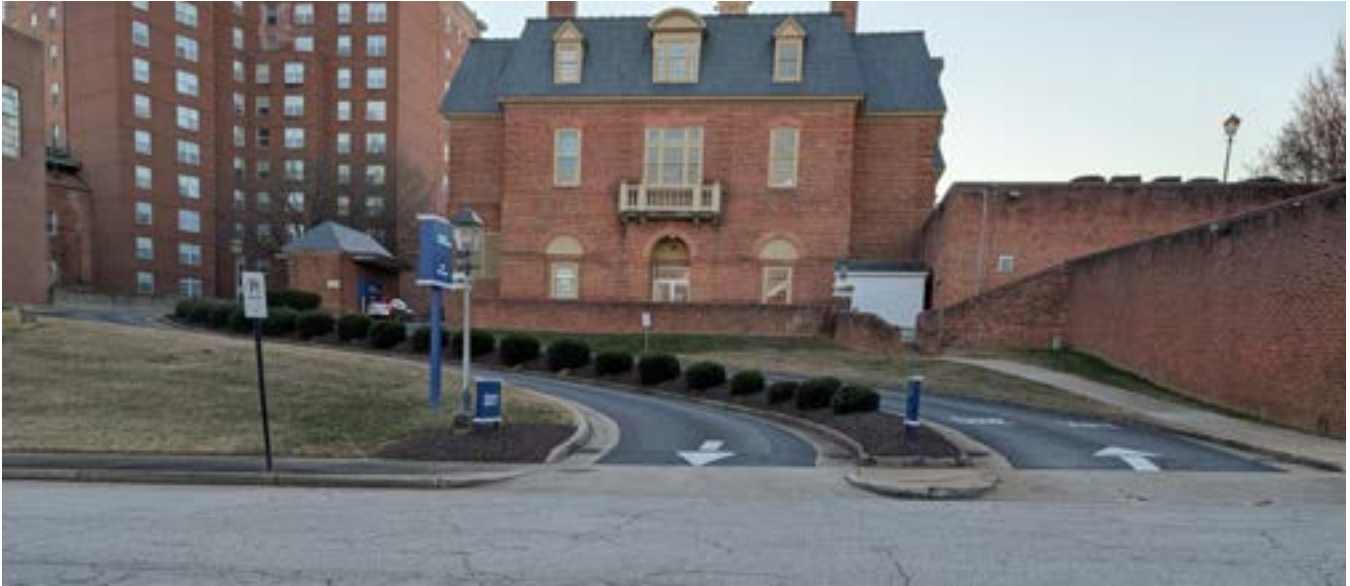
Figure 4.15. The Spring Street access points for First National Bank demonstrates how functional spaces can be aesthetically integrated into public streetscapes.
